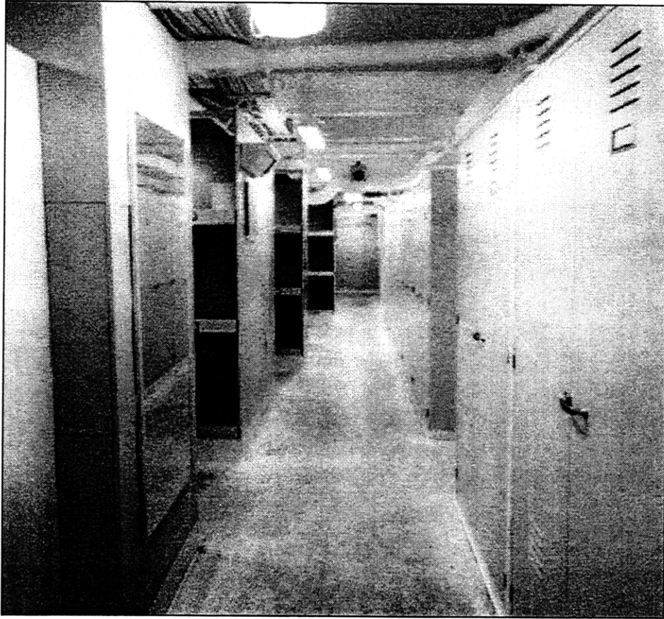
Figure 3-12 – Completed Crew Berthing Space
