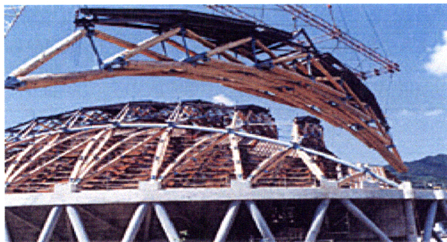
Figure 32: Gujo Hachiman Sogo Sports Center (Takenada Corporation)
