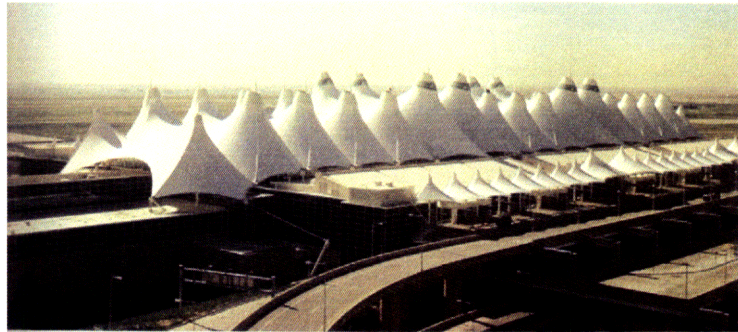
Figure 28 - View of the Finished Fabric Roof (Source: Huntington, 2004)
