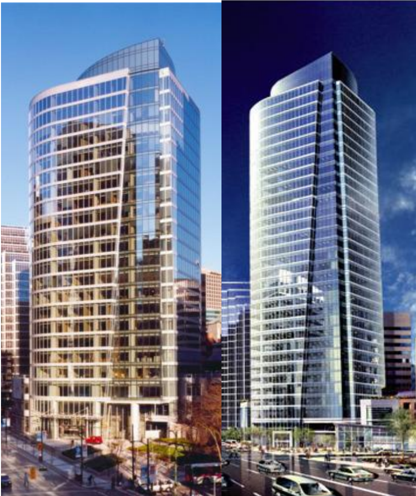
Figure 3. Bentall Five Building in Vancouver Phase 1 (left) and Phase 2 (right) Source: Bentall Capital, 2005 and Pearson and Wittels, 2008
