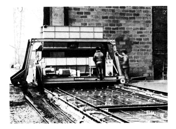
Figure: 34 Spreader receiving the concrete from a transversally traveling storage hopper.
