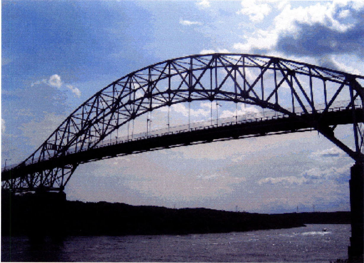
FIGURE 4: SAGAMORE BRIDGE SUPERSTRUCTURE [WWW.BOSTONROADS.COM]
