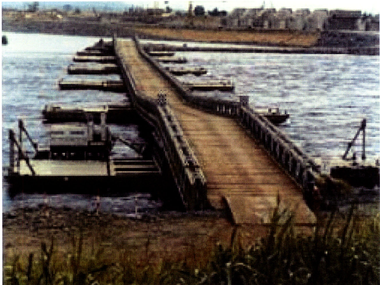
FIGURE 20: BAILEY BRIDGE SUPPORTED BY FLOATING FOUNDATIONS [ WWW.BTINTERNET.COM/~IAN.A.PATERSON ]
