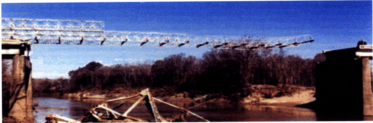
FIGURE 12: BAILEY BRIDGE CONSTRUCTED BY CANTILEVERING OUT [WWW.FHWA.DOT.GOV]
