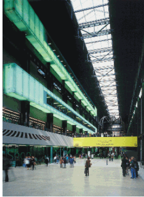
Figure 19 Galleries plugged on the wall inside the Tate Modern
