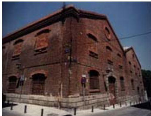
Figure 13 Old Caixa before the transformation
