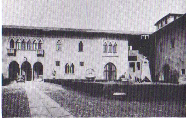
Figure 27 Original facade before the transformation into a museum
