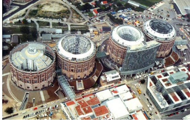
Figure 32 Gasworks after the renovation
