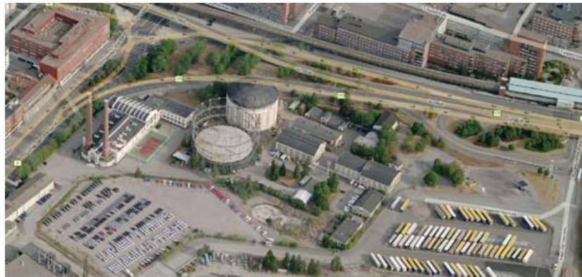
Figure 11 Bird's eye view of the Suvilahti power plant in Kalasatama, Helsinki
