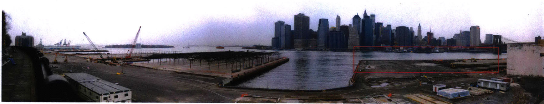
View of the site from Brooklyn Heights (red box denotes site)
