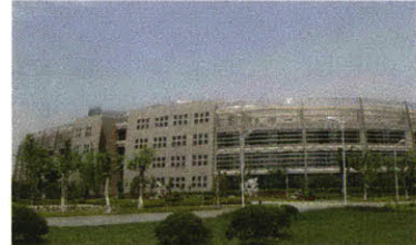
Fig 2.4 College Teaching Building in Minhang District, Shanghai.
