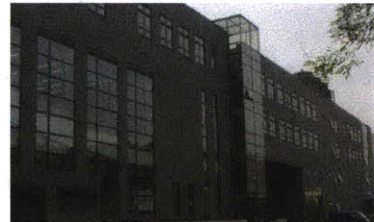
Fig 2.5 College Teaching Building, Beijing
