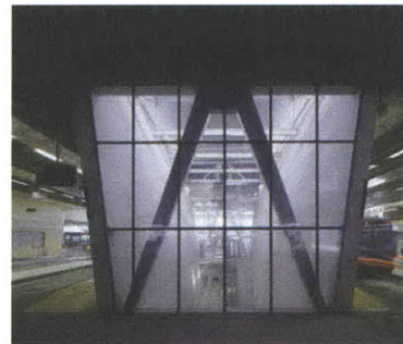
Fig 1.8 Arnhem Central. Underground Car Park. UN Studio. 1996-2010. [Source: Berkel, B. V., & Bos, C. (2002)]
