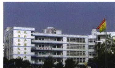
Fig 2.7 High School Teaching Building, Ningbo Province
