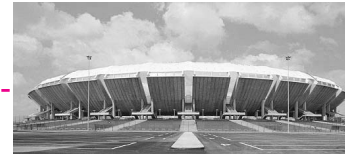
San Nicola Stadium Bari, Italy
