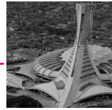
Olympic Stadium Montreal, Canada
