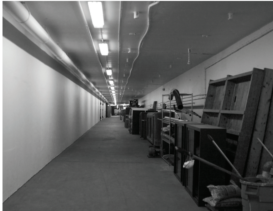
Current view inside the underground bunker looking north.
