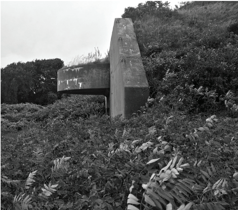
Tunnel through underground bunker (battery number 104).
