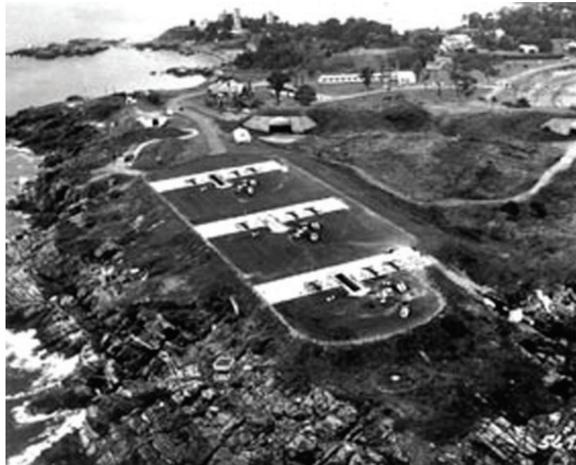
Figure 17: Close-up view of NIKE missile launch area.
