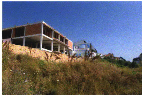
On pedestrian route, looking north
