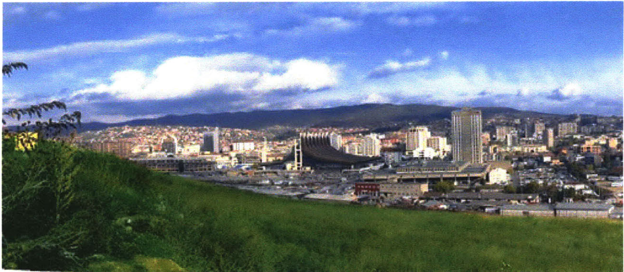
Panorama view from south end of site, looking north, east, and south
