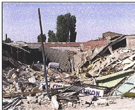
Figure 3.57 Collapsed zone at surface, Istanbul metro (Ayaydin, 2001)
