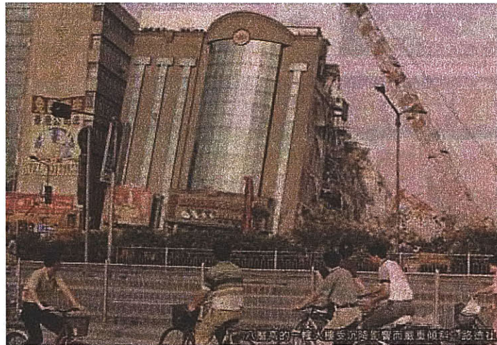
Figure 3.63 Photo at the surface at the site of the collapse at Shanghai metro line 4 (Wannick, 2006)
