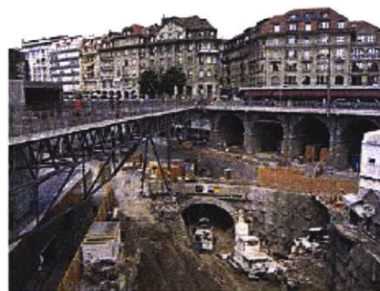
Saint-Laurent tunnel's passage under the 19th Century masonry bridge
