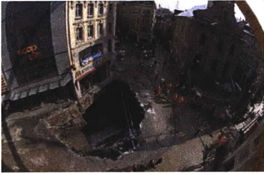
Collapsed area at the surface
