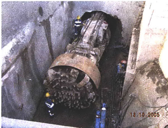
b) TBM used in the excavation
