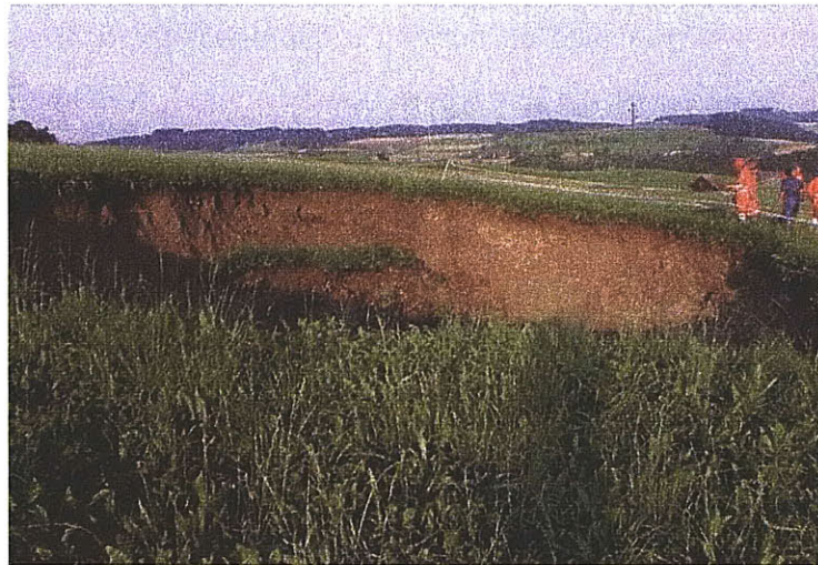
Figure 3.23 Crater caused by a collapse that occurred in the Aescher tunnel, Switzerland (Kovari, and Descoedres, 2001)
