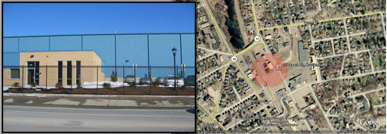
Figure 4-2: Photograph and Air Photograph of the Redeveloped Site in Brockton (DGI Headquarters)
