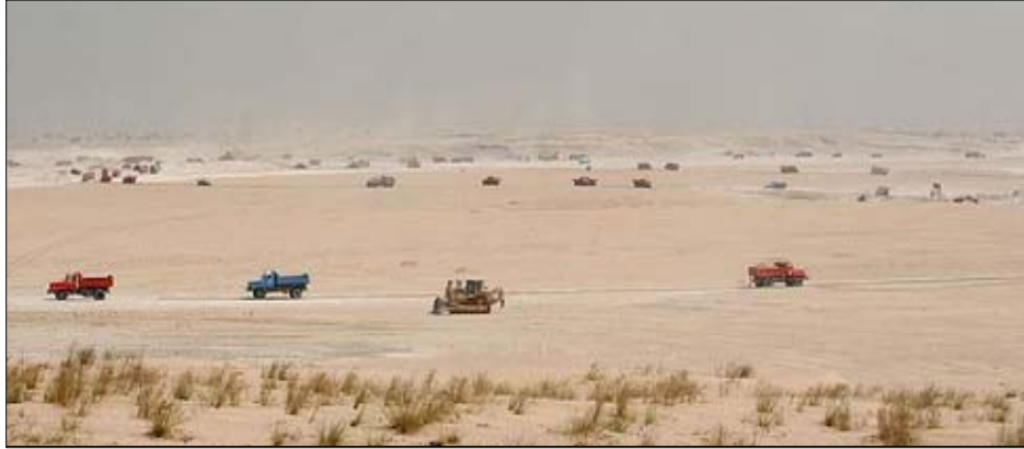
Leveling Dubai's desert for another development (Source: Drew Gardner, Photostream)
