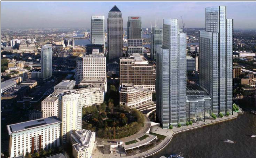
Canary Wharf (Source: Davenport Wind Engineering, Canada)
