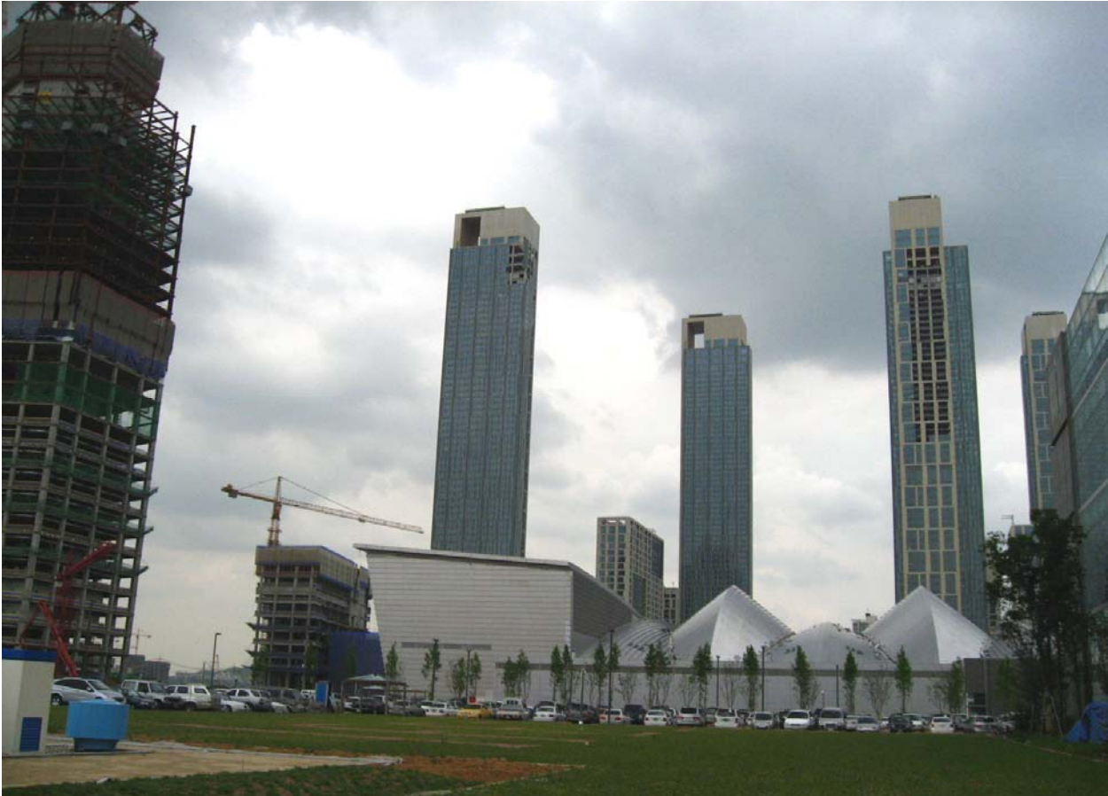
Figure 5 Site Photo on June 3, 2008
