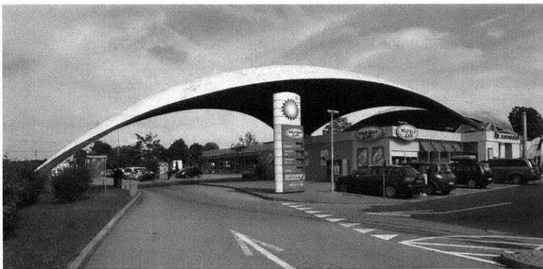
figure_7 Motorway Service Station, Deitingen Sud, 1968, Heinz Isler
