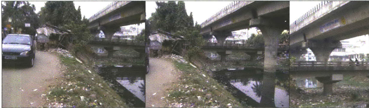
Metro Piercing the channel
