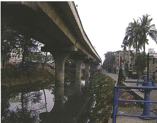
Fig 1.3: Metro columns Source: The author
