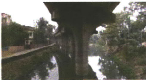
Fig 3.18: Image of Metro piers on the channel
