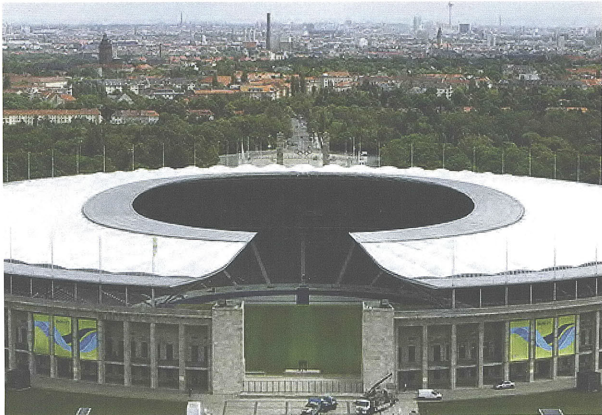
The new roof on the Olympiastadion as seen from above.
