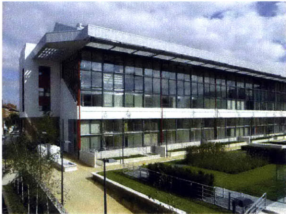
Image of apartments and garden Photo Credit: www.highburysquare.com
