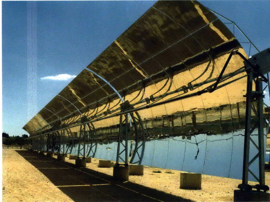
Figure 1: Array of parabolic troughs in the Negev desert of Israel. A parabolic trough uses a parabolic reflector to concentrate the sun's rays into a central focus line directed at the receiver, a tube filled with a working fluid that collects the sun's energy as heat. The receiver is often a pipe filled with oil that is circulated through a steam generator to produce electricity [7].
