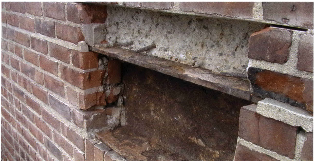
Figure 44: Destructive Test Cut of Masonry Façade
