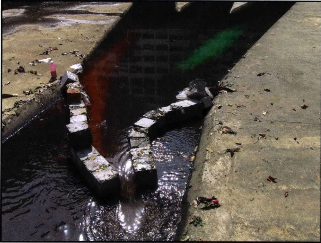
Figure 3.2: Induced hydraulic jump to promote mixing of three confluent channels at upstream end of attenuation study.
