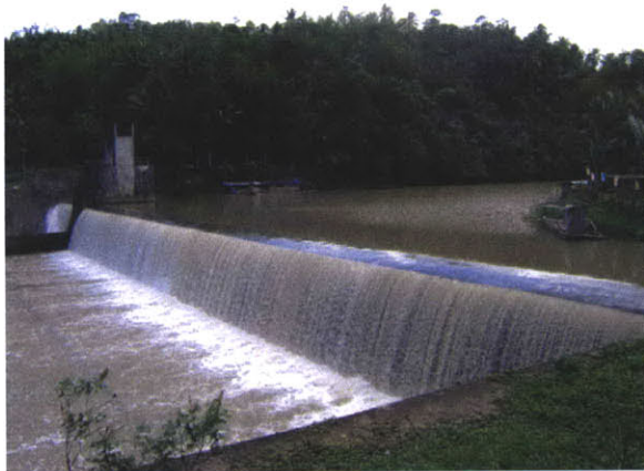
Figure 6: Current Irrigation Dam
