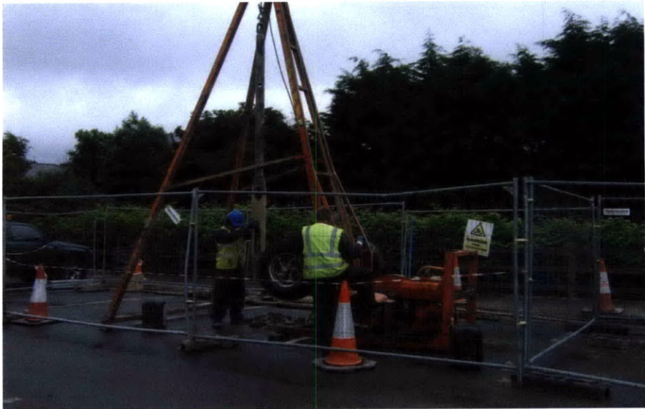
Figure 2-35: Shell and auger for site investigation boreholes
