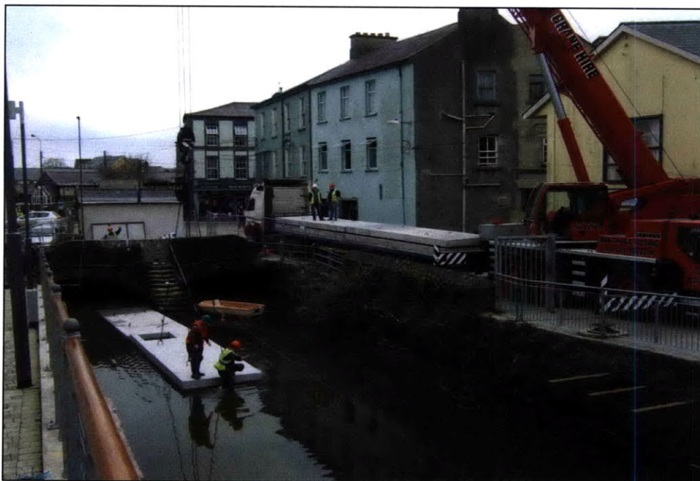
Figure 2-33: Addition of kentledge over tunnel
