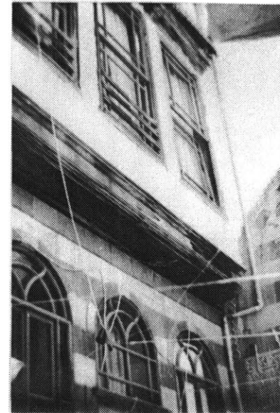
Fig II.16: A view of one of the courtyards after renovation.
