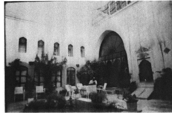
Fig IV.4: View of the courtyard in Nijad's house after renovation. Note how the liwan has been glazed and forms now part of the interior of the house.
