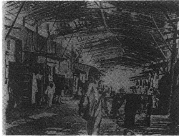
Source: Ronald Lewcock and Zahra Freeth, Traditional Architecture in Kuwait and the Northern Gulf , London, 1978
