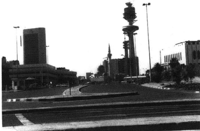
[Fig. 5] New telecommunication tower dwarfs minarets
