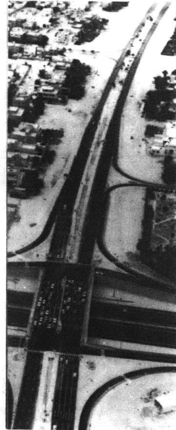
[Fig. 22] Expressway isolating residential neighborhoods Source: Ministry of Information, Kuwait: Facts and Figures, 1988
