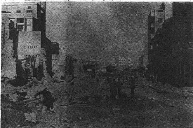
[Fig. 49] Demolition for implementing CBD Plan
