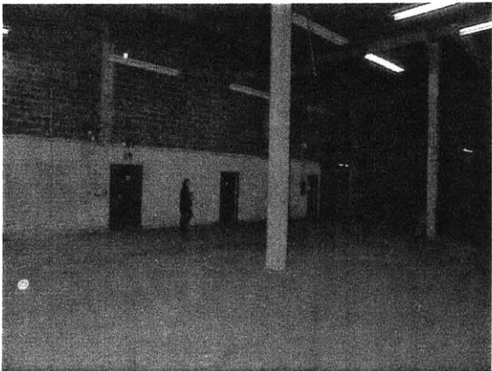
as-built condition: upper floor
