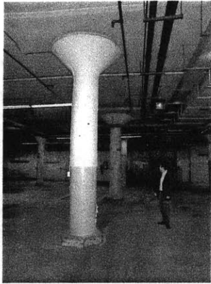
as-built condition: basement
