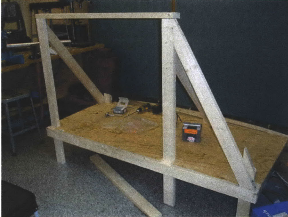
Figure 22: Structure with completed door frame, floor, and supports.
