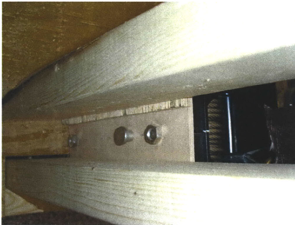
Figure 25: View showing bolts and mounting plate of the winch.
