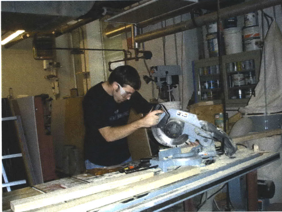
Figure 16: Demonstration of wood sections being cut.
