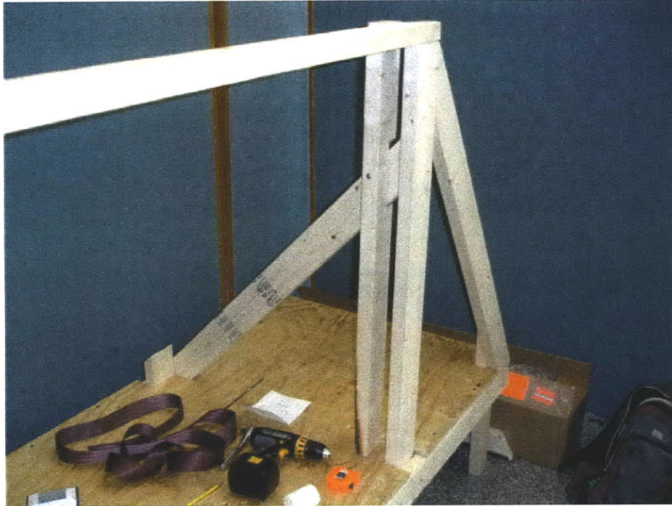
Figure 23: Additional support board attached to door frame, floor, and side support.
