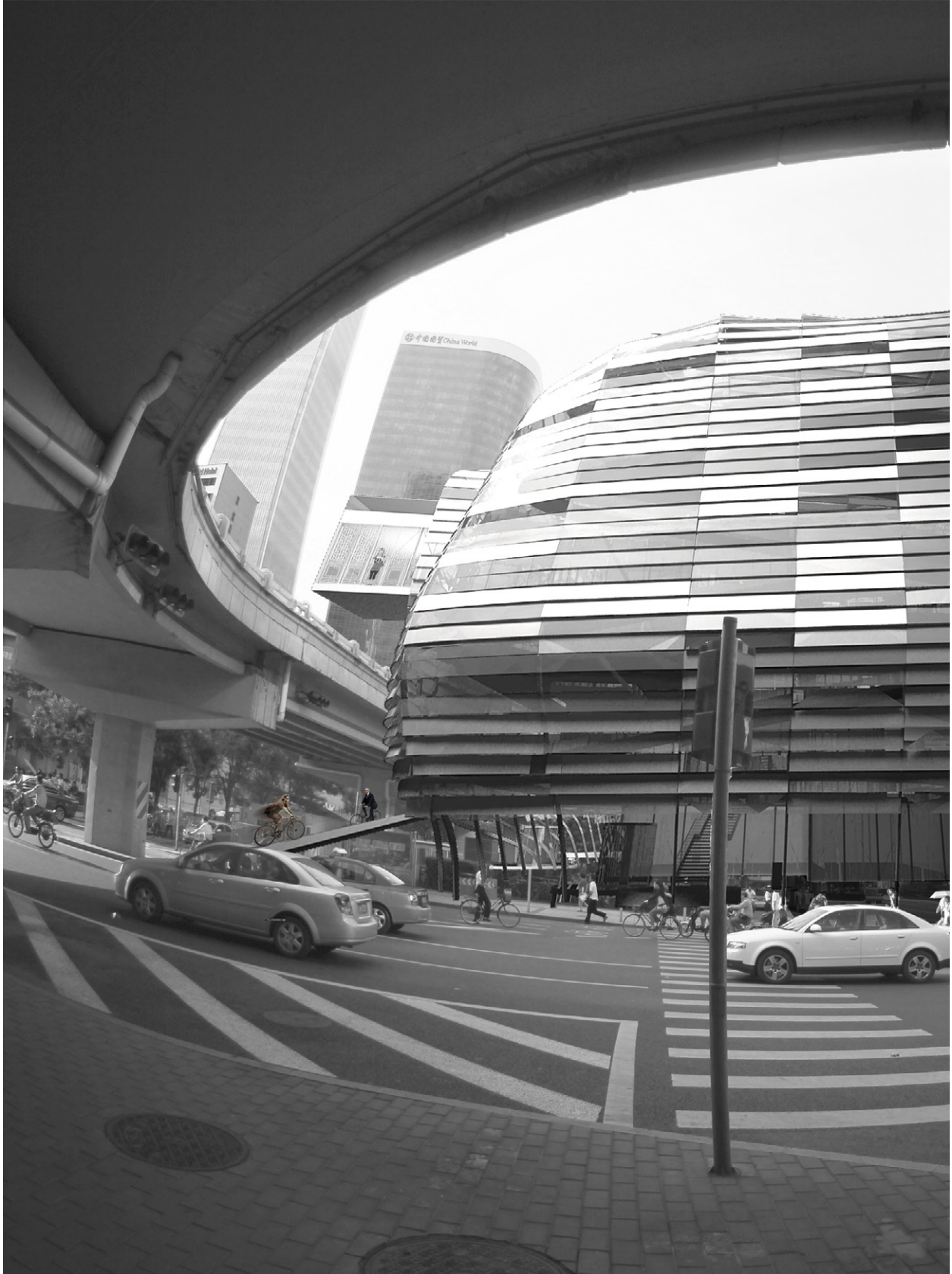
View of open lower level, facade above and connecting ramps
