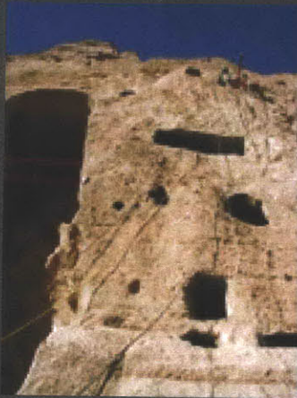
The smaller caves were also reinforced, since they have gone through a fair amount of wear from the trafficking of the Taliban, and the armies.
