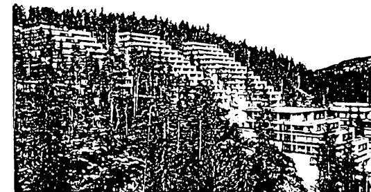
Friis. The residential complex in Ullernaasen, near Oslo.
