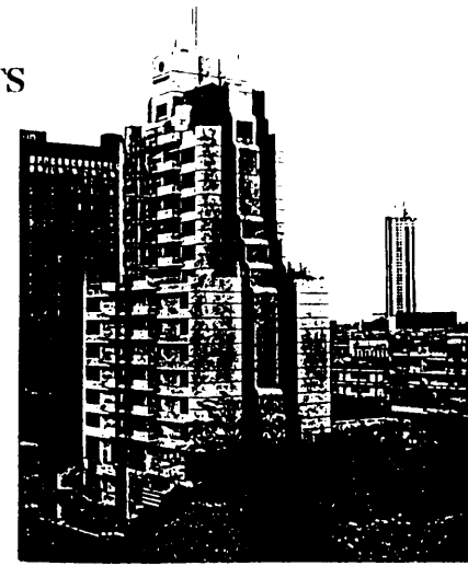
Sithakorn Condominium: 1984 Chidlom Rd., Bangkok
