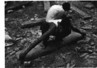
Fig.82. Worker replacing paving.
