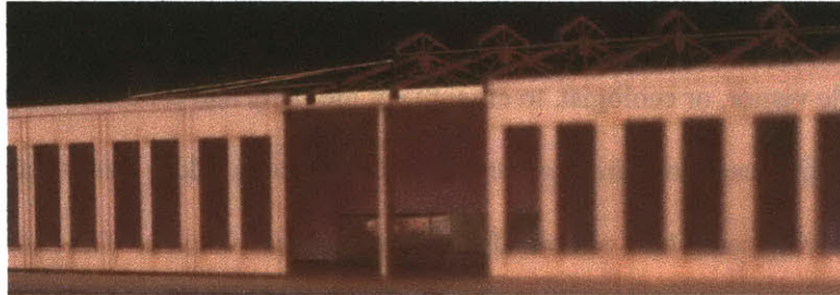
VIEW OF EAST FACADE AT CONNECTION POINT TO VERDADUCT
