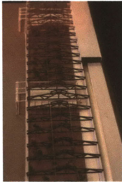
AERIAL VIEW OF ROOF
