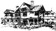
27 F. H. Van Dusen House, Washington, Connecticut, by Potter and Robertson, 1879-82. ( American Architect , 1882)
