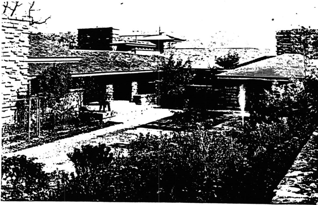
44. Taliesin I, Spring Green, Wisconsin, 1911. Roofs and Court.
