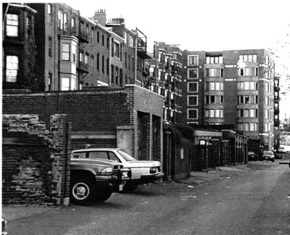
Typical alleyway in block structure
