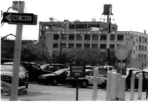
Abandoned factory buildings downtown, Nature has reclaimed the roof. July, 2002.
