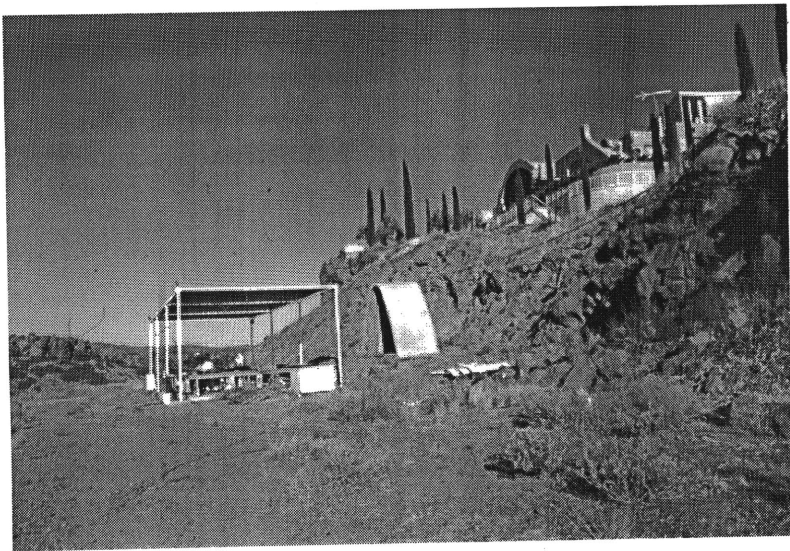
The Silt casting site. Main access level is \sim +16 feet.
