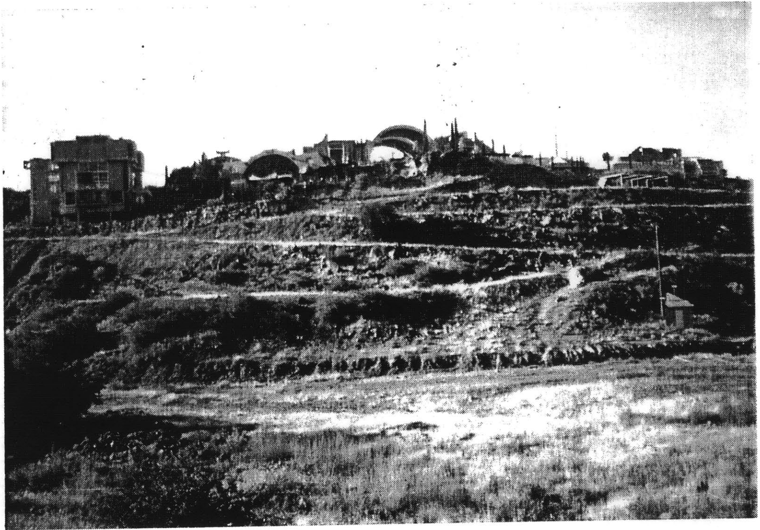
The horizontality of the ground
