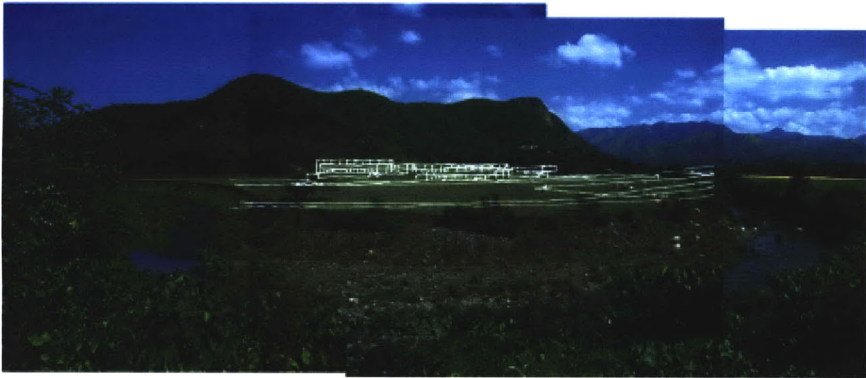
View from the road looking west. The building is perceived as a series of planes which are flattened out in the distance.
