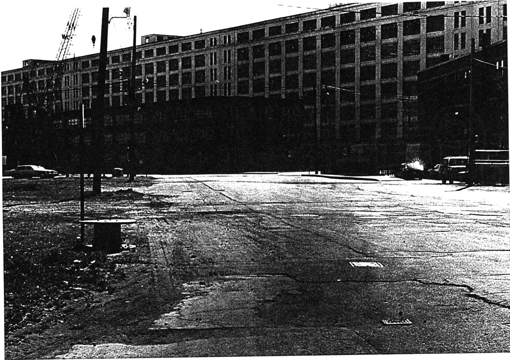
Figure 4.1 A stretch of roadway in Boston's Marine Industrial Park prior to redevelopment. (photo courtesy of BMIP)
