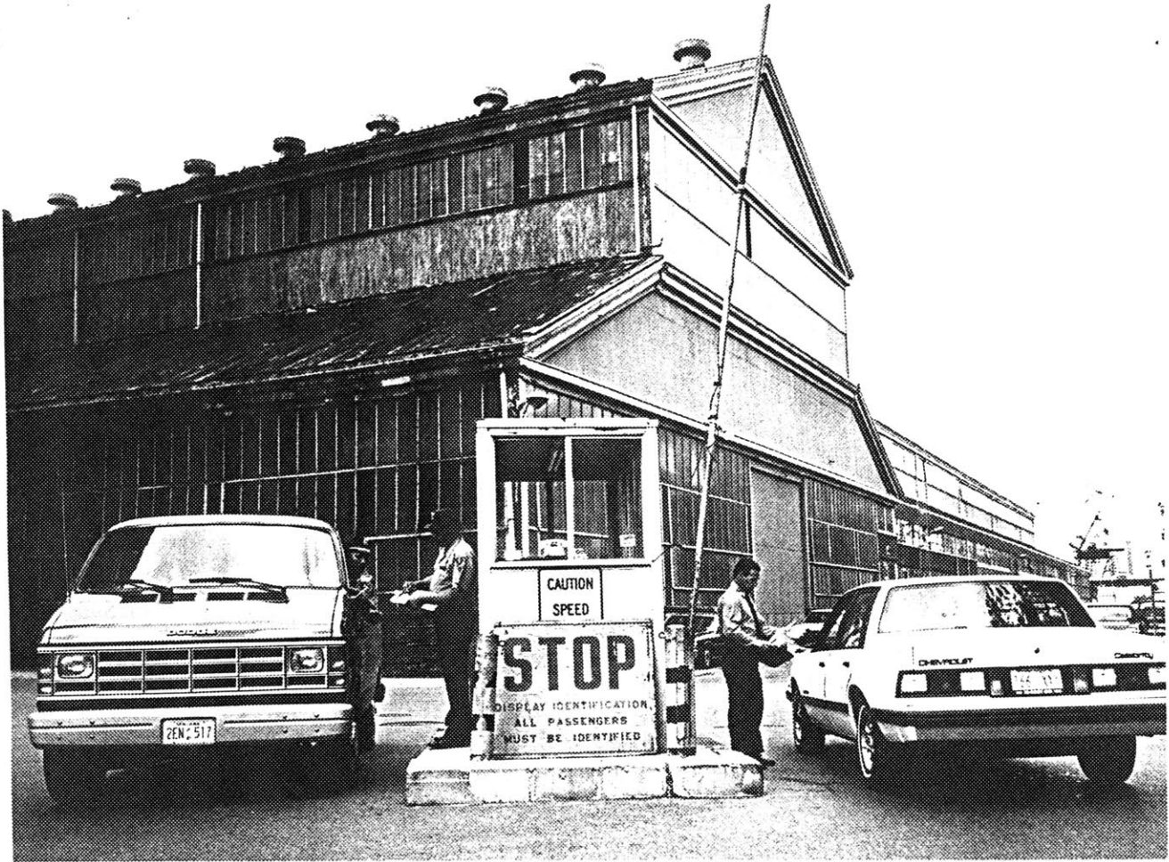
Figure 2.5 The BNY operates its own security force of 60. Vehicles are monitored as they both enter and exit the site. (photo courtesy of BNY)
