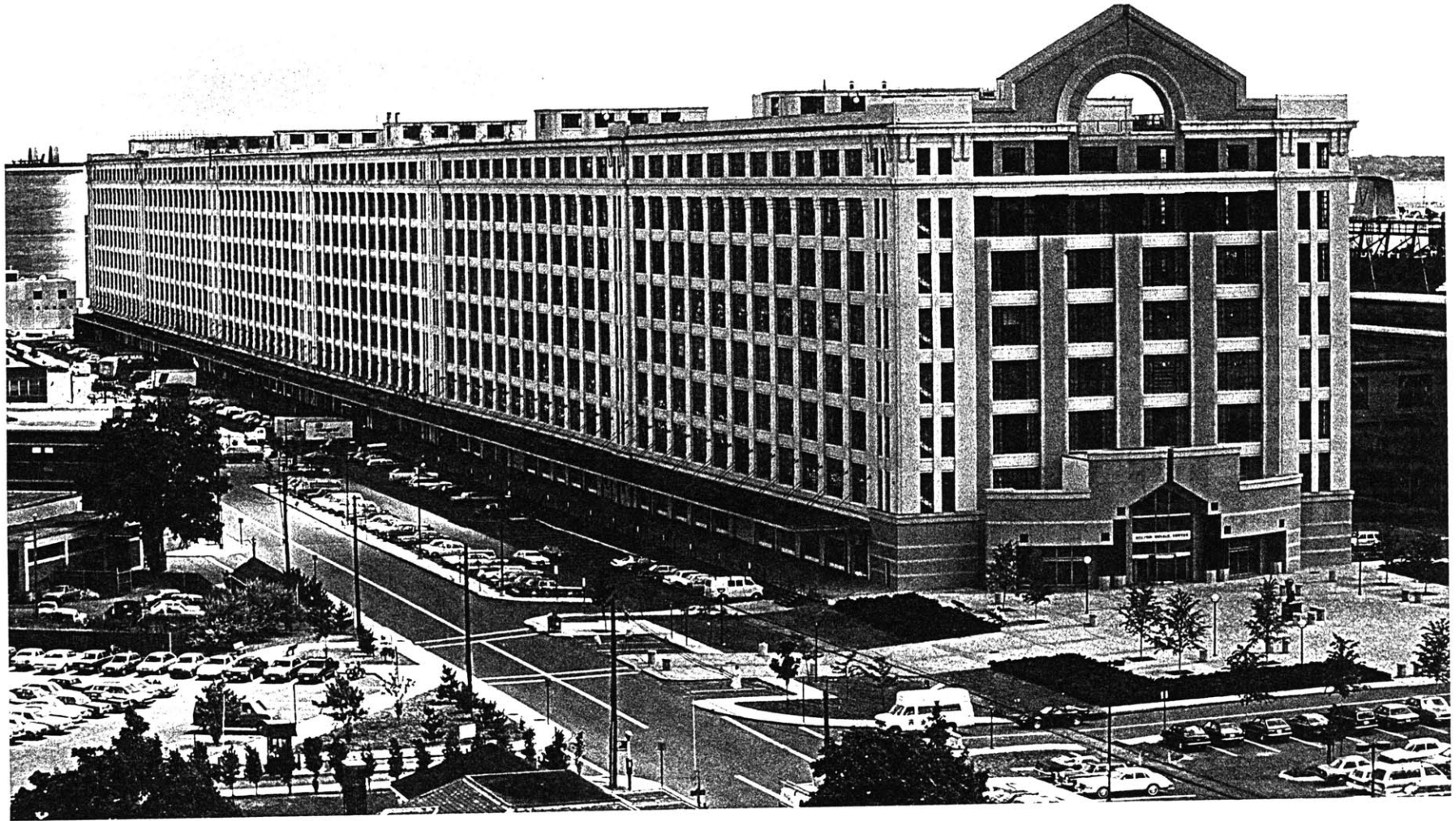
Figure 3.7 The BMIP's Building 114 -- eight stories tall, a third of a mile long. (photo courtesy of BMIP)
