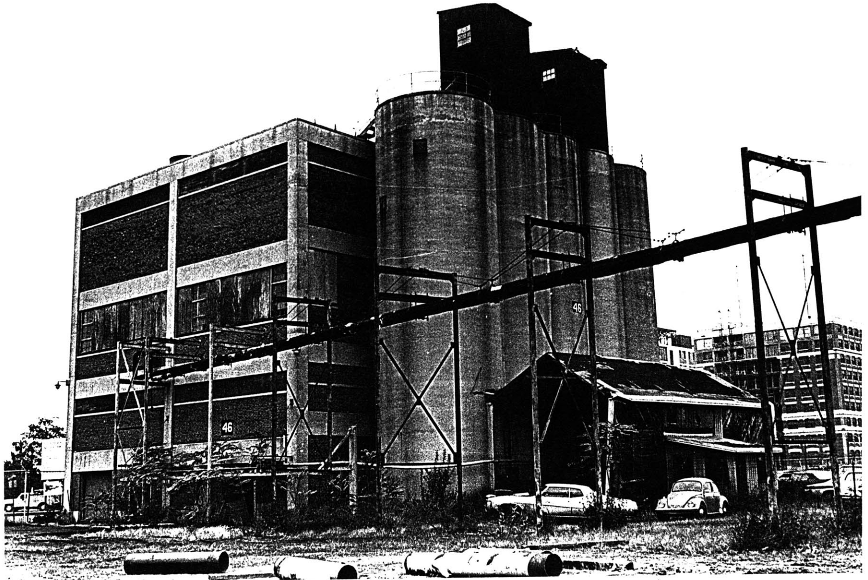
Figure 1.3 The Boston Marine Industrial Park's Building 46 - a former cement works- is a typical derelict structure.(photo courtesy of BMIP)
