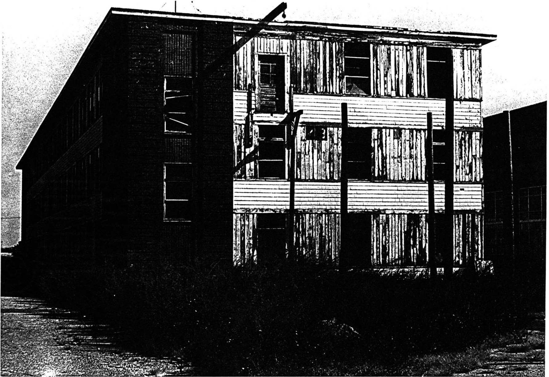
Figure 1.2 Building 48 of the Boston Marine Industrial Park: an example of industrial dereliction. (photo courtesy of BMIP)
