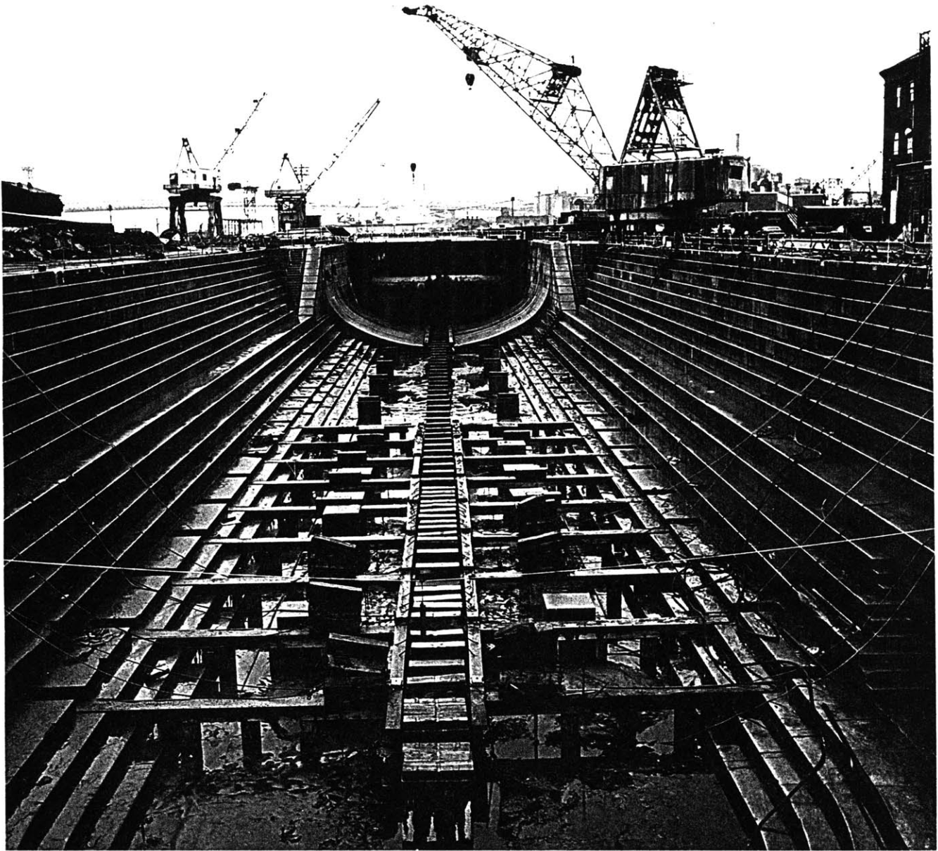
Figure 4.5 Marine facilities, like this drydock at the BNY, should be an integral parcel of the redevelopment strategy, and can generate revenue at the beginning of the process. (photo courtesy of BNY)
