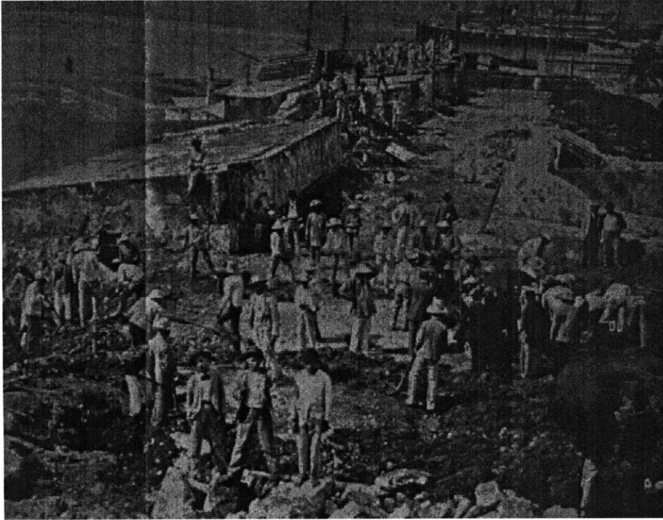
Figures 42 - Demolition of the wall.
