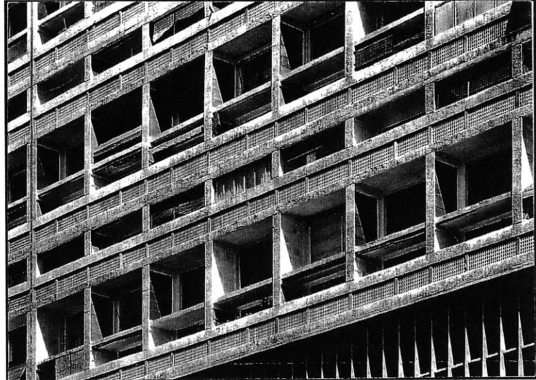
Fig. 7.59 Le Corbusier's, 1945-52, Unité d'habitation à Marseille Rigid use of a proportioning system. The rigid layout of the structural frame did not allow much variation
