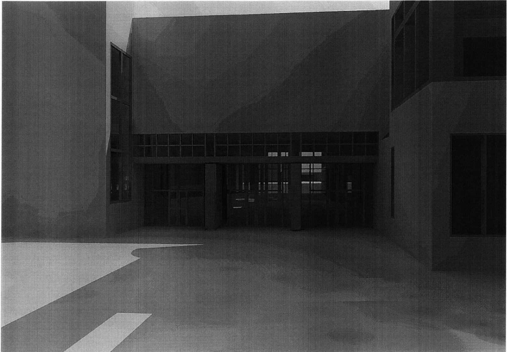
View of entry plaza demonstrating entry experience under solid compressive element towards light and water.
