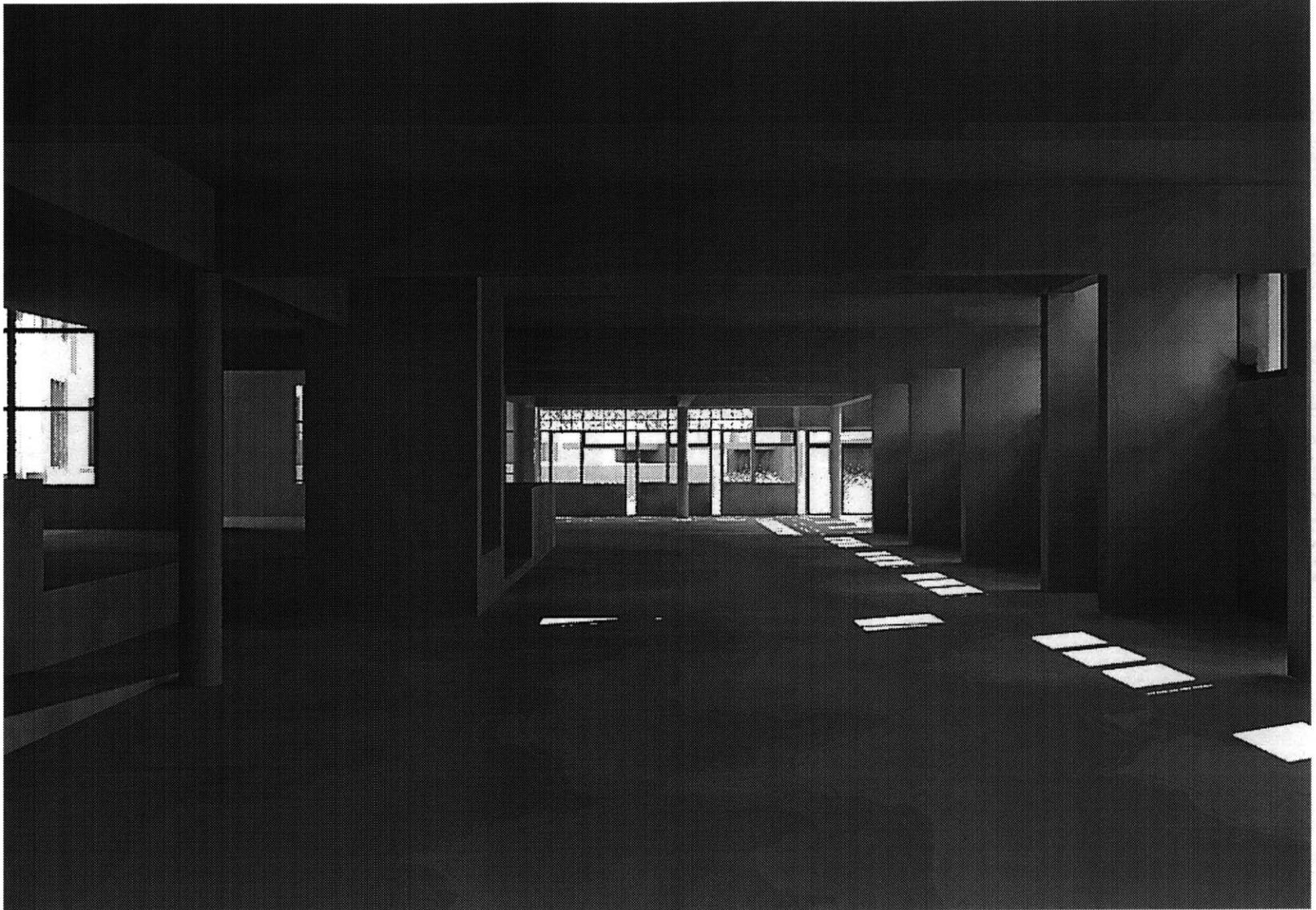
View South to corner.
