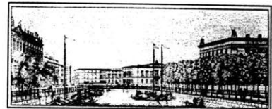
Perspective view by Schinkel of the Neue Packhof and the Museum, 1834. From Mackowsky.
