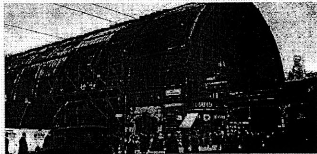
View of the post-war destruction to the station.
