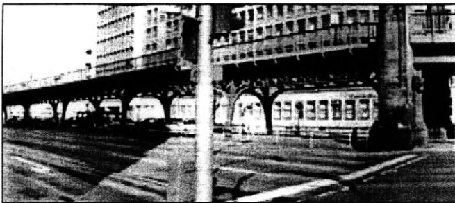
View of the elevated railway looking at the opposite direction.
