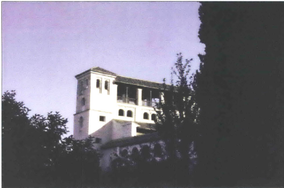
Fig. 2.16 Two stories were added to the northern pavilion of the Generalife in 1494
