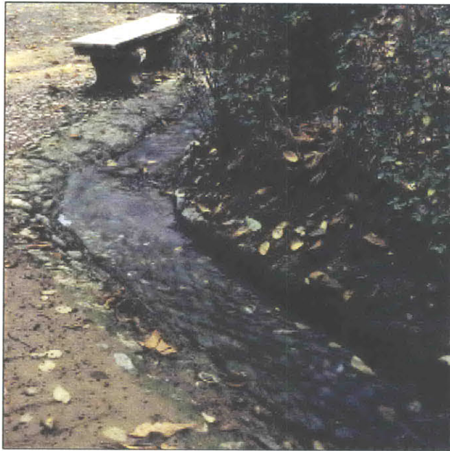
Fig. 3.5 Detail of ornamental irrigation channels in the Alhambra Wood in the Poplar Grove
