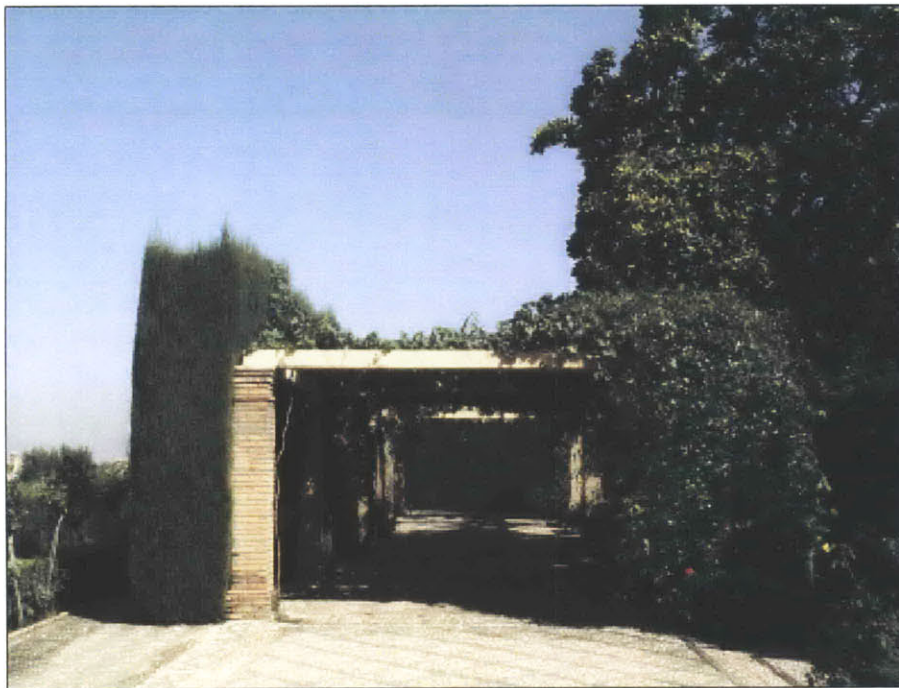
Fig. 2.41 Trellised walkway overlooking the Alhambra of the 1930's garden of the Generalife
