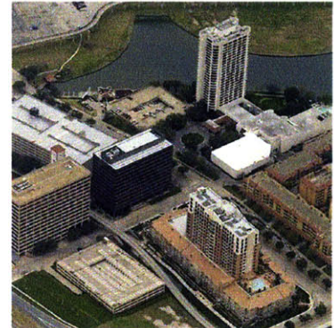
Figure 02.08 Las Colinas Urban Center High-rise towers in the Las Colinas development in close proximity to DFW, surrounded by single family homes.
