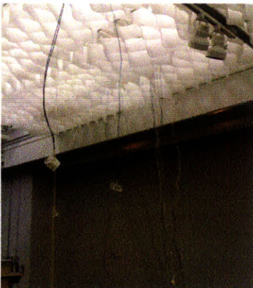
Figure A1.08 Wiring Wiring being installed in Gund Hall.
