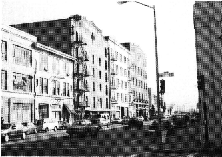
Warehouse wall in the north-south direction
