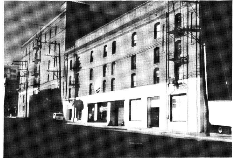
Warehouse wall in the north-south direction
