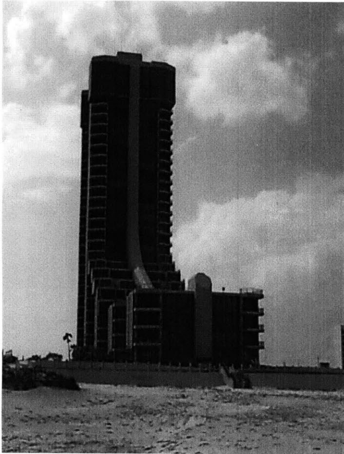
Figure 5.6 High-rise condo with bulkhead.
