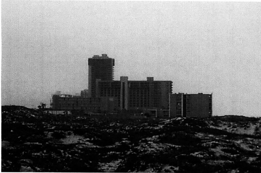
Figure 5.7 Shoreline development in natural sand dune area.
