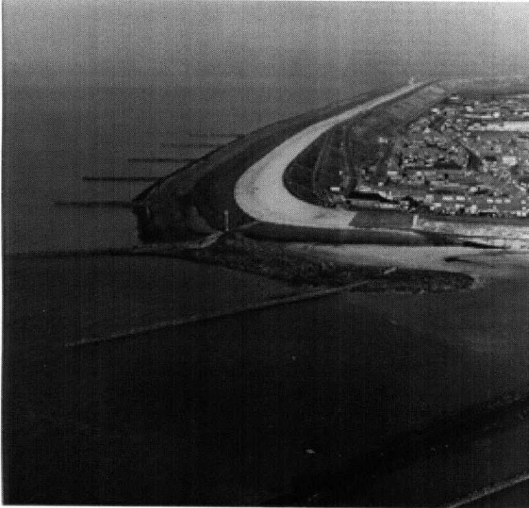
*Scientific American, March 1997: Sea dikes protect low-lying areas of the Netherlands from the ocean, which rises above the land in many places. The Dutch government must maintain hundreds of kilometers of dikes and other flood-control structures on the coast and along riverbanks.
