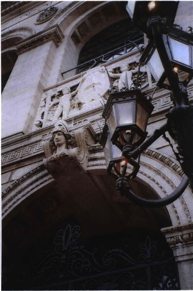
Top Left: Entrance and light fixtures, McKim Building.
