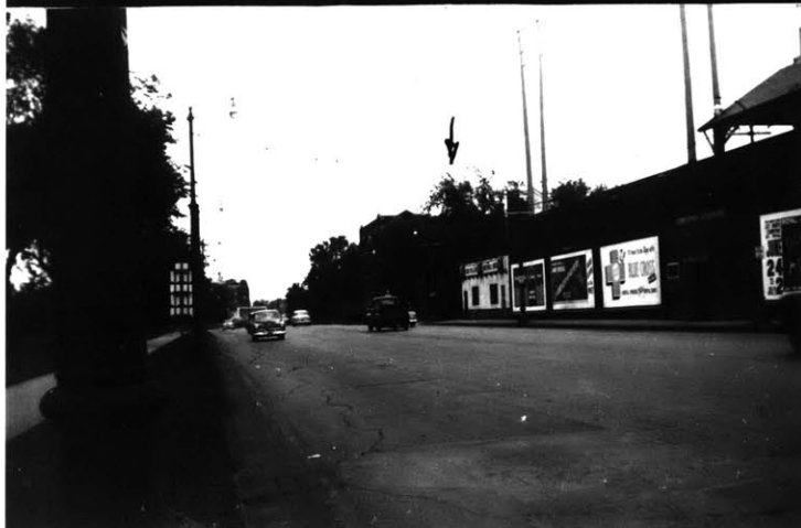
Looking South down Osborne Street Site marked below arrow
